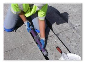
Figure 2. Inserting dowel bar assembly into slot (Photo courtesy of Jeff Uhlmeyer, Washington State DOT).
